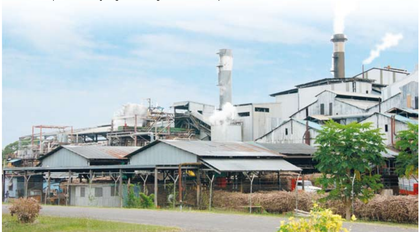
Lautoka Mill in crushing operations
